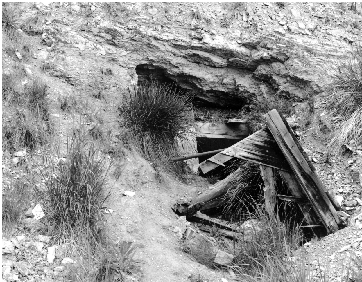
Figure 66. Caved Home Canyon Mine portal, June 24, 1996. Photo by the author.
